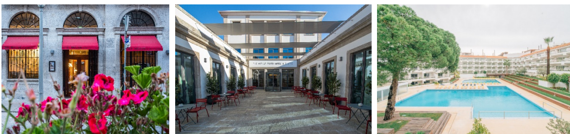
Picture 6: The House Ribeira Hotel, The Artist Porto Hotel & Bistro and Aqualuz Lagos.
